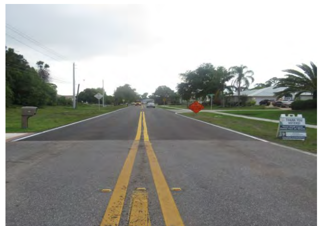
Tulip – Completed paving project with sign
