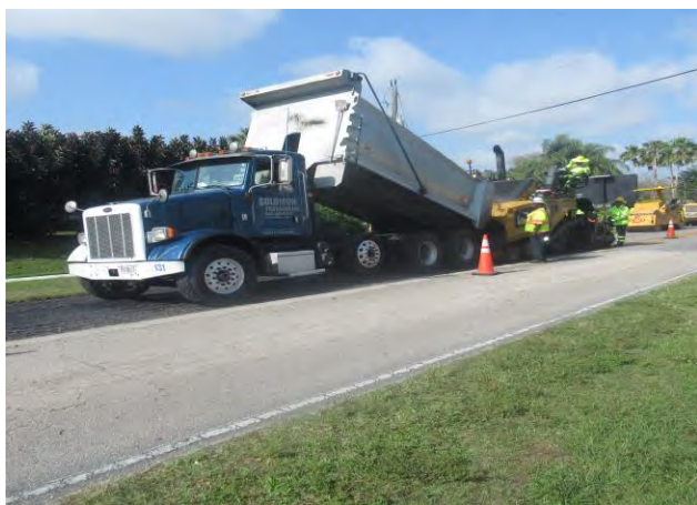
Tulip – Paving in progress
