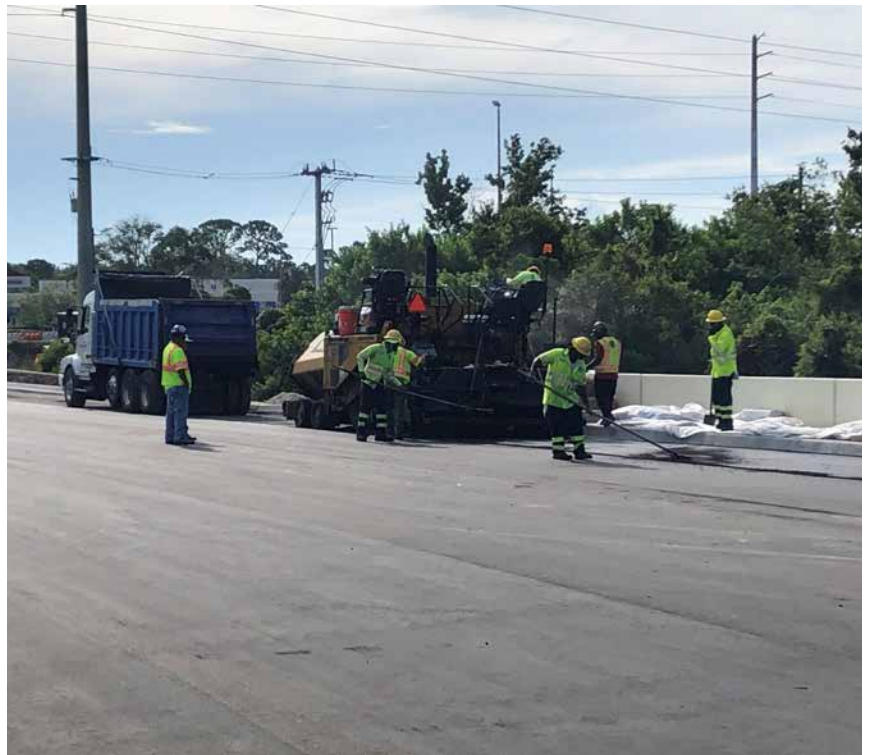
Asphalt on the bridge approaching east side of the project.
