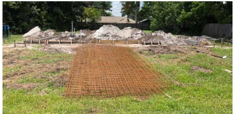
SE Asbury Lane: Construction has begun.
