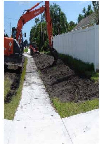
Paar Dr. (PSL/Savona) Grading side swale
