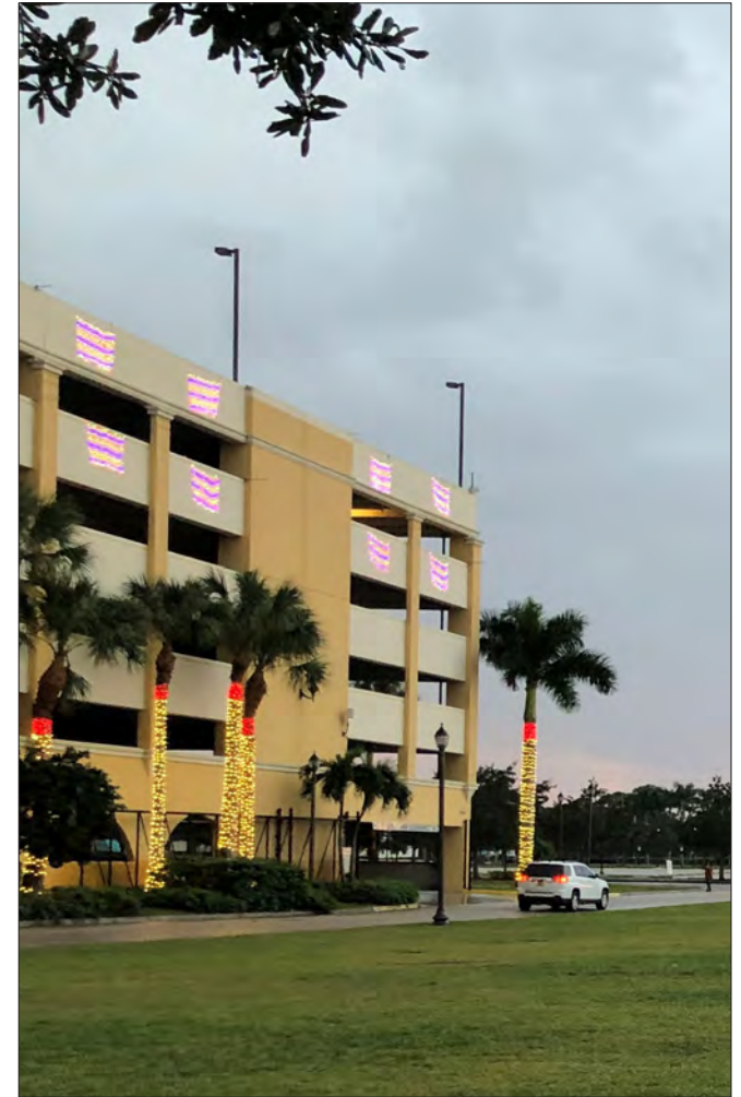
Figure 104 Image of the existing 900-space Garage 1.
