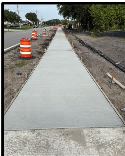
Lakehurst Sidewalk Construction
