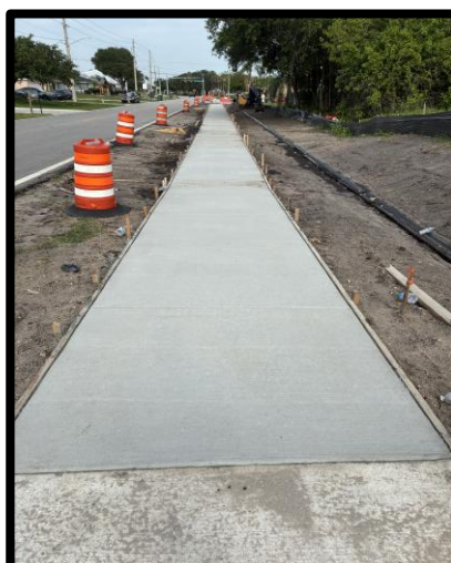
Lakehurst Sidewalk Construction
